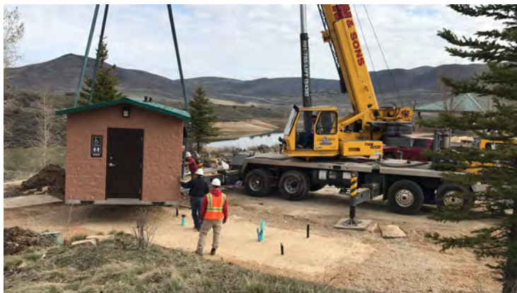
New restroom at Keetley Group Campsite.
