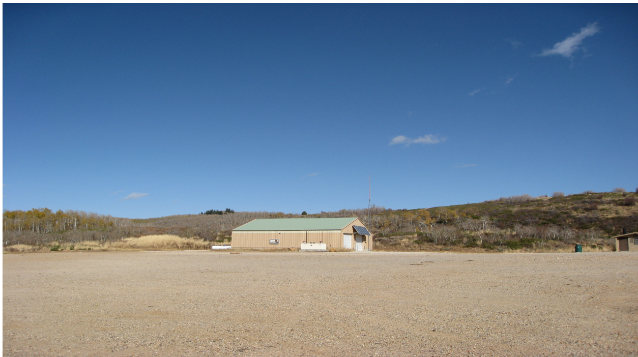
Monte Cristo State Recreation Area Maintenance Building
