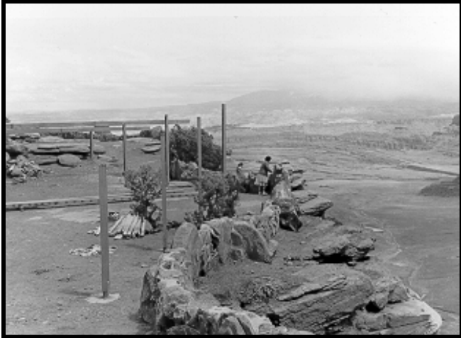
Viewpoint Shelter Under Construction 1961
