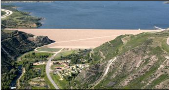
Photo 1-3: Jordanelle Dam looking upstream
